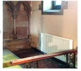
8. The heating will be on its own electrical supply. In addition, as part of the overall project, two new double sockets will be installed on each of the three walls. These will be positioned to take account of refreshment preparation, use of projectors and audio equipment, cleaning and other items needing power. The contractor has also agreed to use front plates for the sockets more in keeping with the building than the white plastic ones currently installed.
