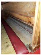
The floor is mainly of wood and carpeted in the sanctuary, aisle and entrance area. Beneath the pews and choir stalls it is bare wood and there are electric tube heaters, covered by guard nets, fastened to the floor below the pews. The central aisle is a more solid surface (stone or concrete) but has been covered with carpet for many years. There were originally heating pipes in channels with grills over them along the aisle but these have been removed.
